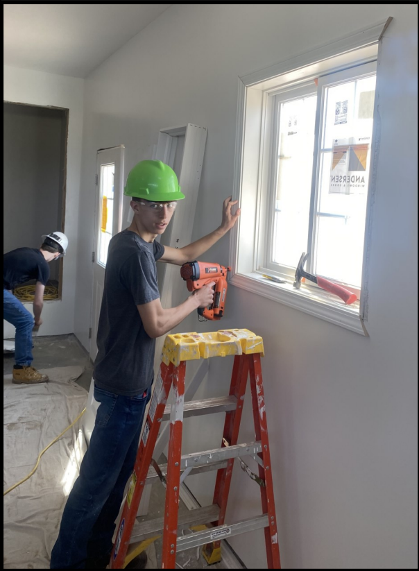
Jayden Wrusch (O) installing window casings.
