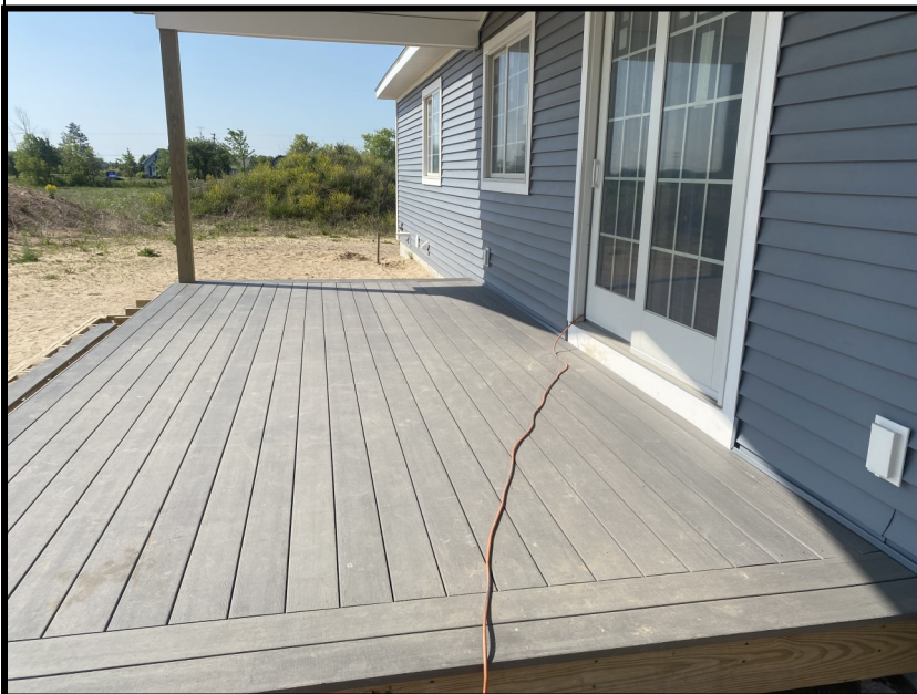
(bottom right) Installation of the flooring.
