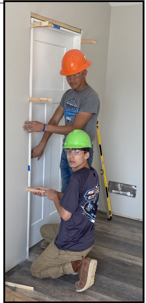
(above) Eli Murphy (WP) and Dylan Cockrell (WP) installing a door.
