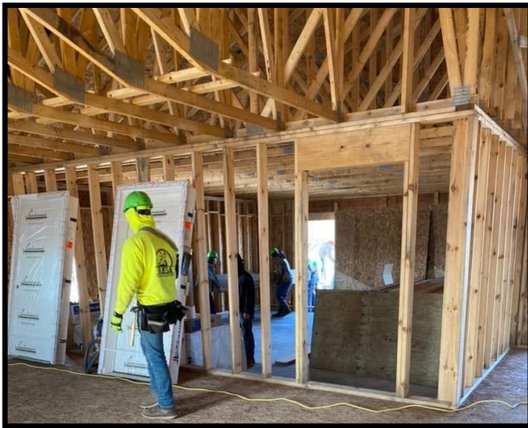
(above) Students working during the in-house skills competition installing windows and doors.
