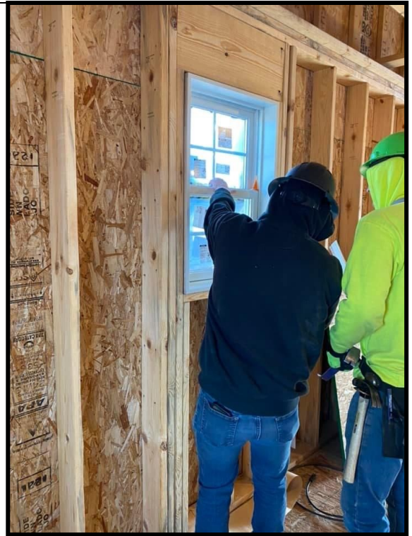
Students installing windows during their in-house skills competition.
