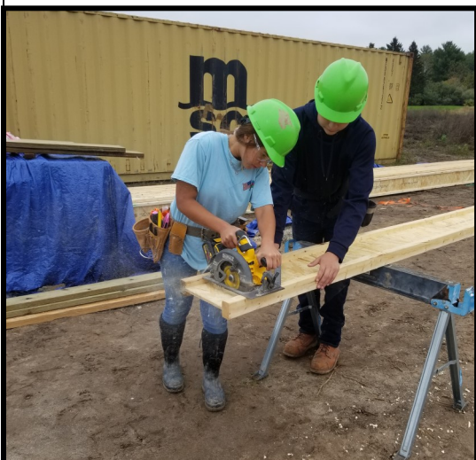
(left) Tawas students; Alia Abbott and Devin Bellinger, cutting floor joists.
