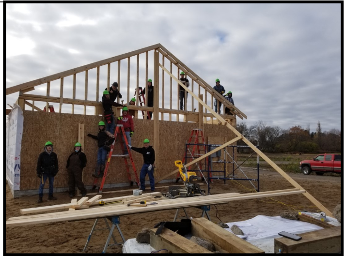
(above) Morning session students posing after setting their first truss successfully.
